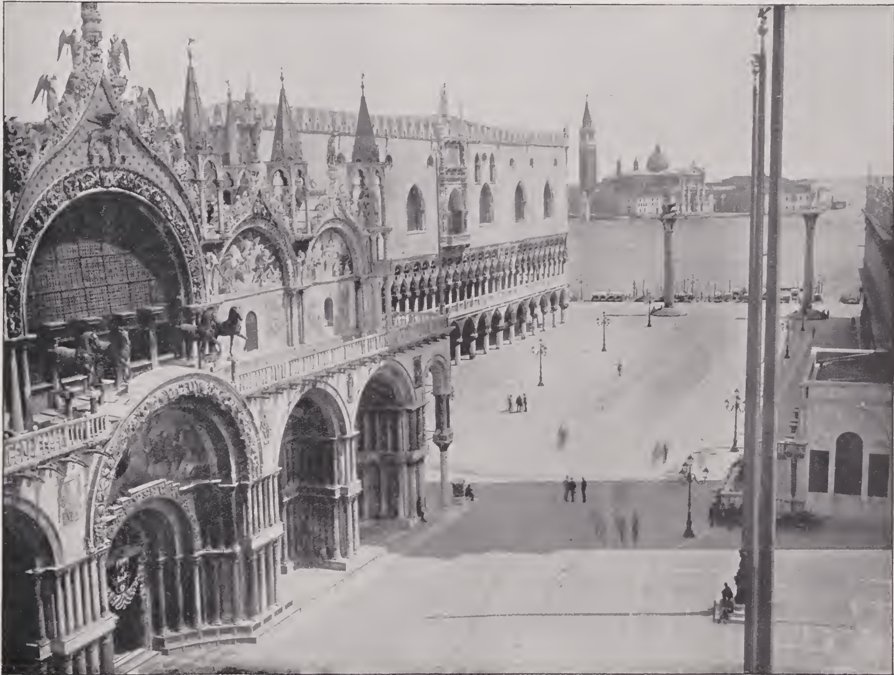
CATHEDRAL OF ST. MARK, VENICE, ITALY.—Facing the piazza of St. Mark, which is in the heart of Venice, and the grand focus of attraction, rises the magnificent Cathedral of St. Mark, decorated with almost oriental splendor. The building dates back to the tenth and eleventh centuries, and portions of the materials used in its construction have been brought from almost every country in Europe. The ceiling of the interior is richly adorned with mosaics in the form of various noted paintings. Behind the High Altar repose the remains of St. Mark, while further back stand four spiral columns said to have belonged to the Temple of Solomon. The building to the right is the Ducal Palace.
